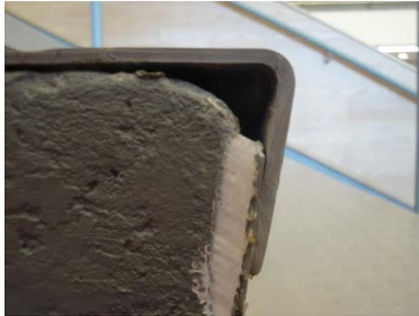
A stair tread that is laid as shown in the picture above will break at the nosing due to repetitive flexing.
