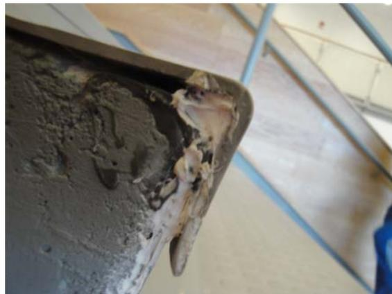
Make sure that the internal part of the nosing is filled properly with NC-888 epoxy caulking to prevent any flex.
