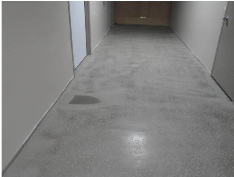
The floor is repaired where it is justified
